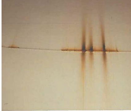
Corrosion along interior shell weld seam.
