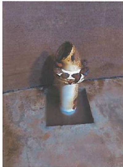
58. Corrosion on piping in sump.
