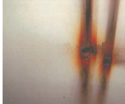
Corrosion on interior shell.
