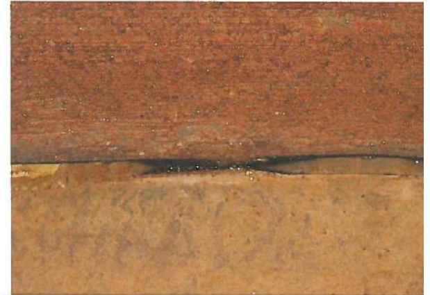
54. Voids in material along shell-to-floor connection.
