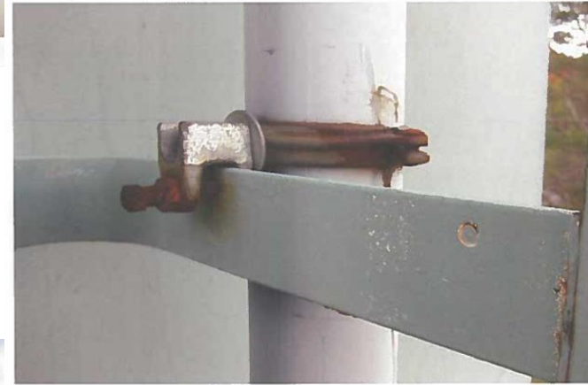
22. PVC pipe bolted to ladder safety cage.
