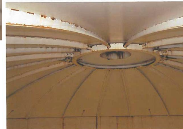
38. Corrosion on roof stiffeners.
