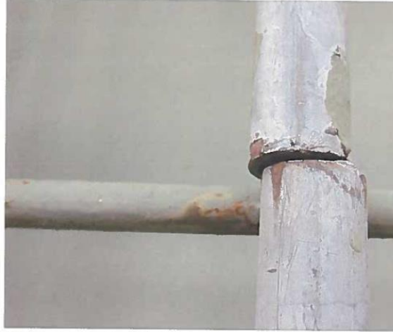
23. Misaligned notched-tubular rail sections.
