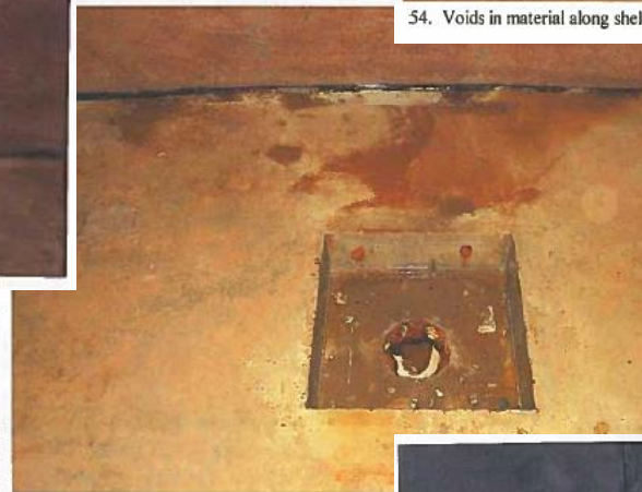
58. Corrosion on piping in sump.
