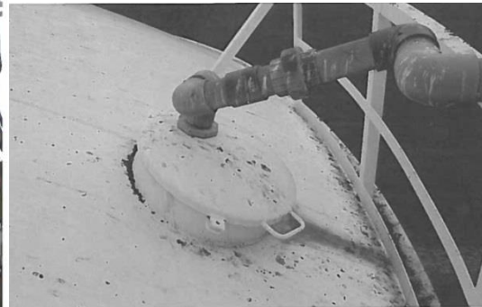
5. Pipe attached to hinged roof manhole cover.
