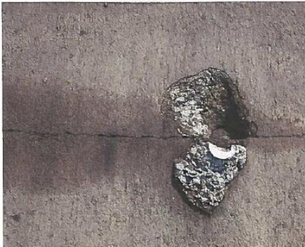
33. Spalling and cracking in roof.
