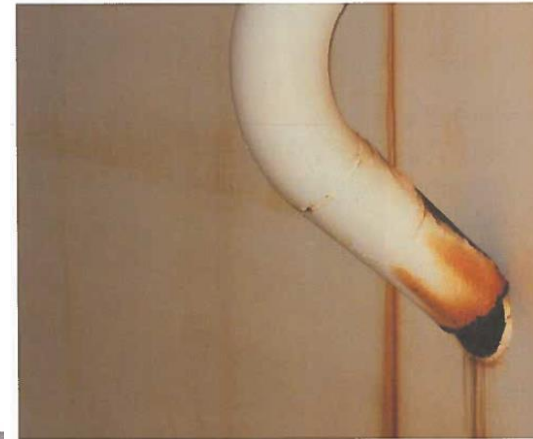
44. Overflow pipe no longer attached to shell.
