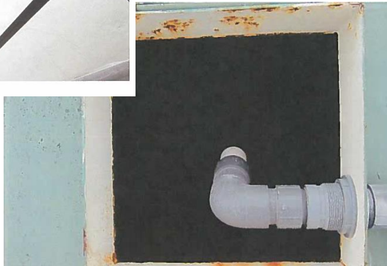
29. Piping extending into roof manhole.
