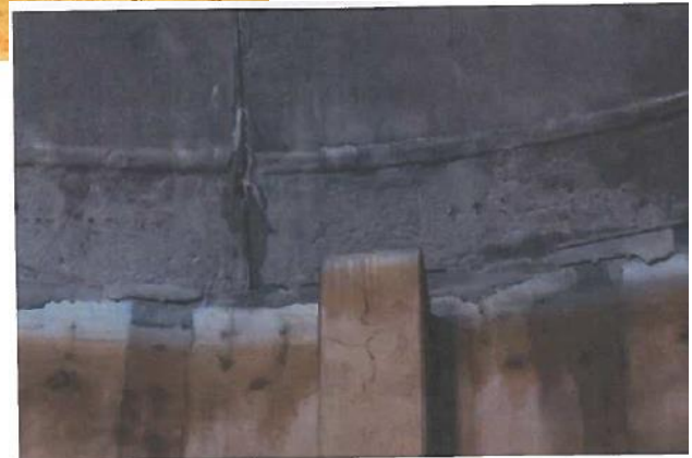
43. Concrete encasing overflow inlet.
