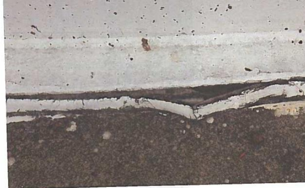
14. Peeled sealant along grout and bottom plate.
