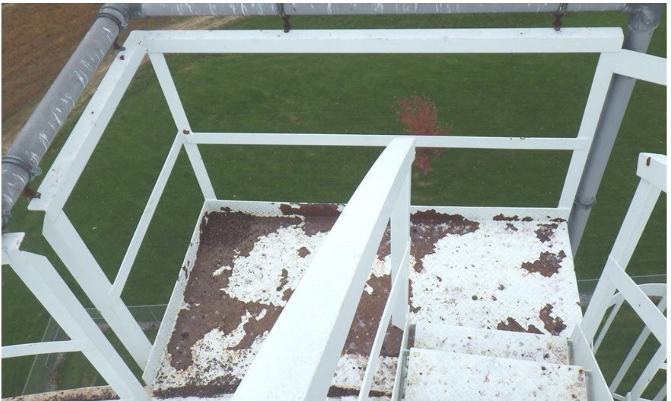
34. Platform at roof.
