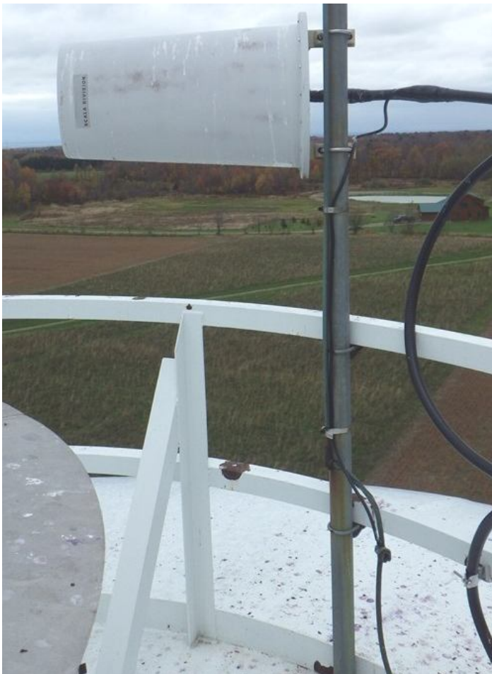
44. Antenna near center of roof.
