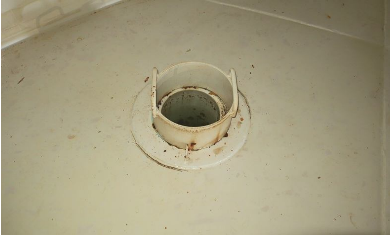
64. Outlet pipe with removable mud ring.
