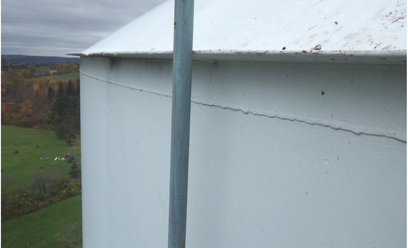
32. Conduit at top of shell.
