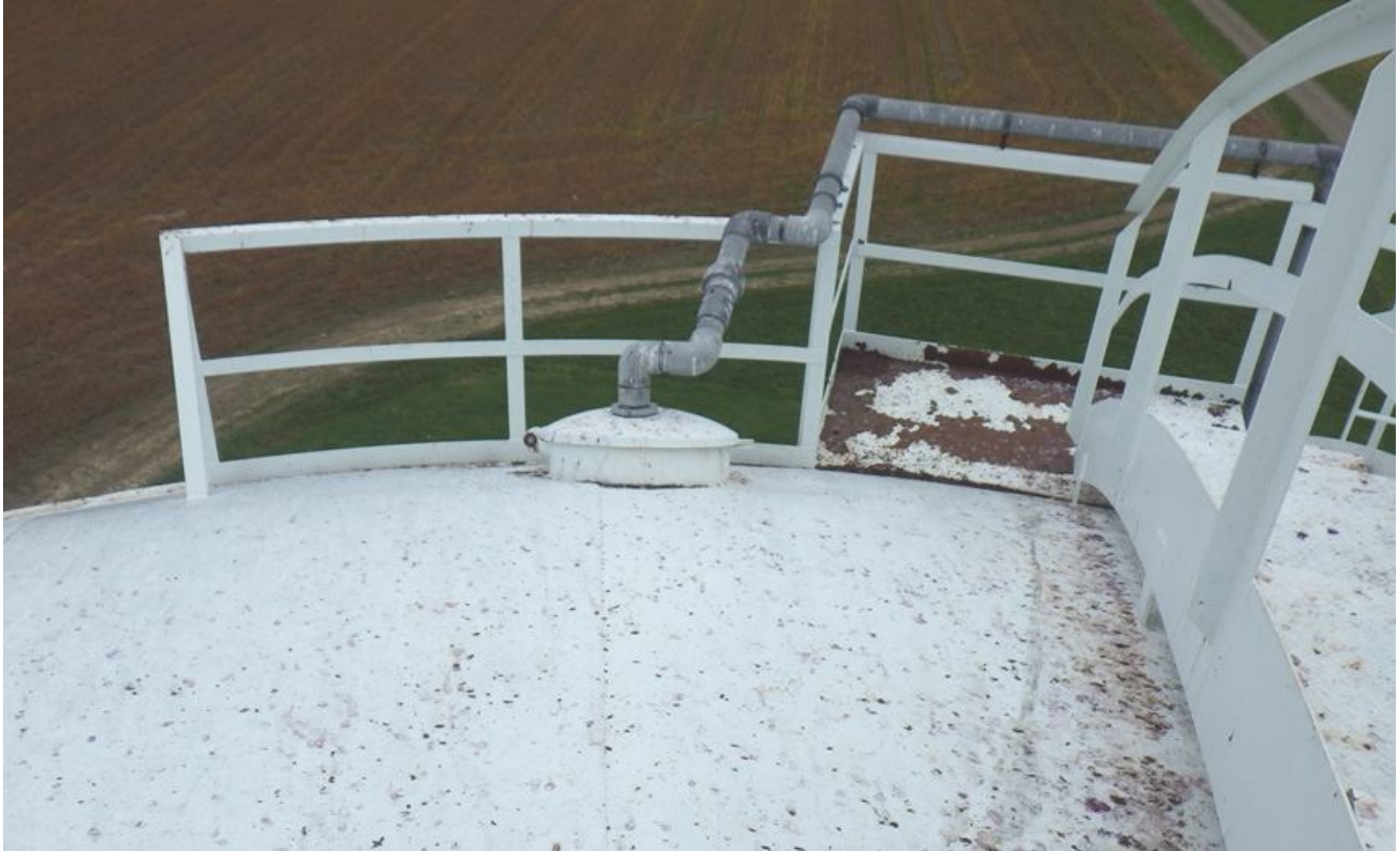
36. Roof safety railing, platform, stairs, and pipe attached to hinged roof manhole cover.
