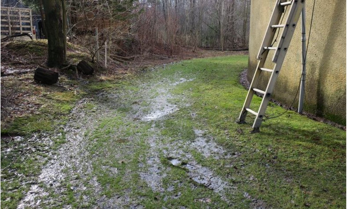
6. Water standing around tank.
