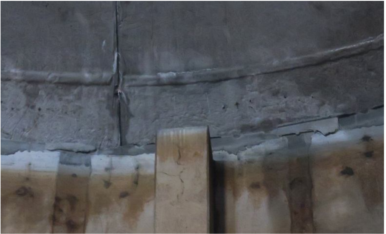
43. Concrete encasing overflow inlet.
