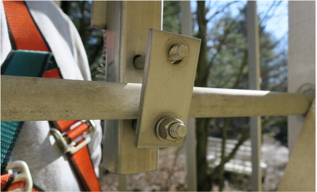
21. Safe-climbing device bracket not equipped with washer and nut.
