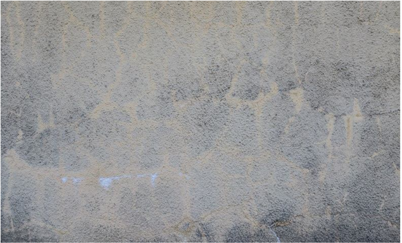
17. Efflorescence on shell.
