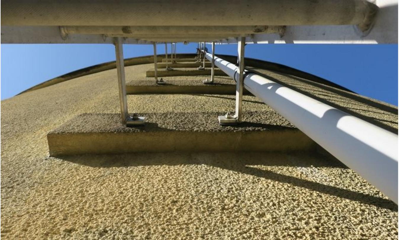
20. Exterior ladder, brackets, and conduit.
