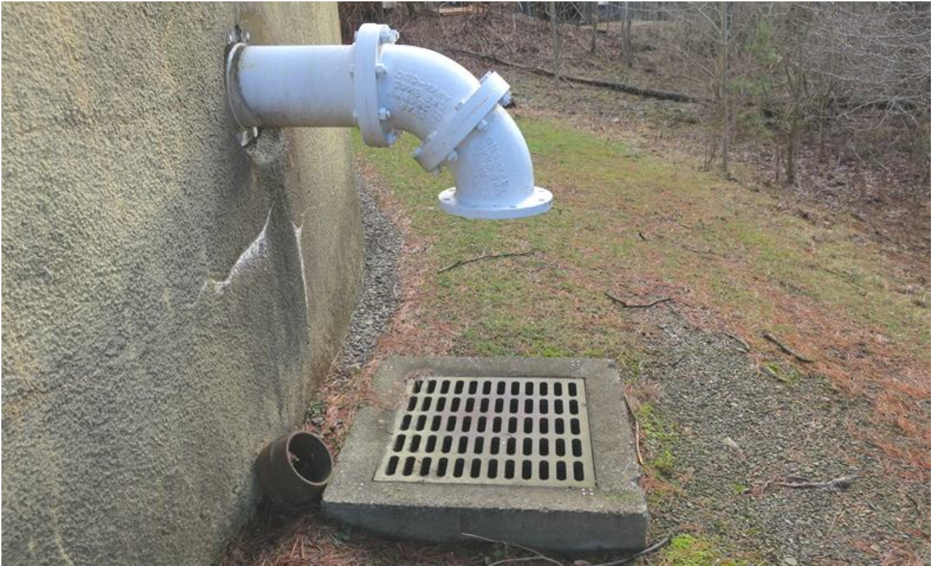
9. Overflow pipe discharge above drain basin.
