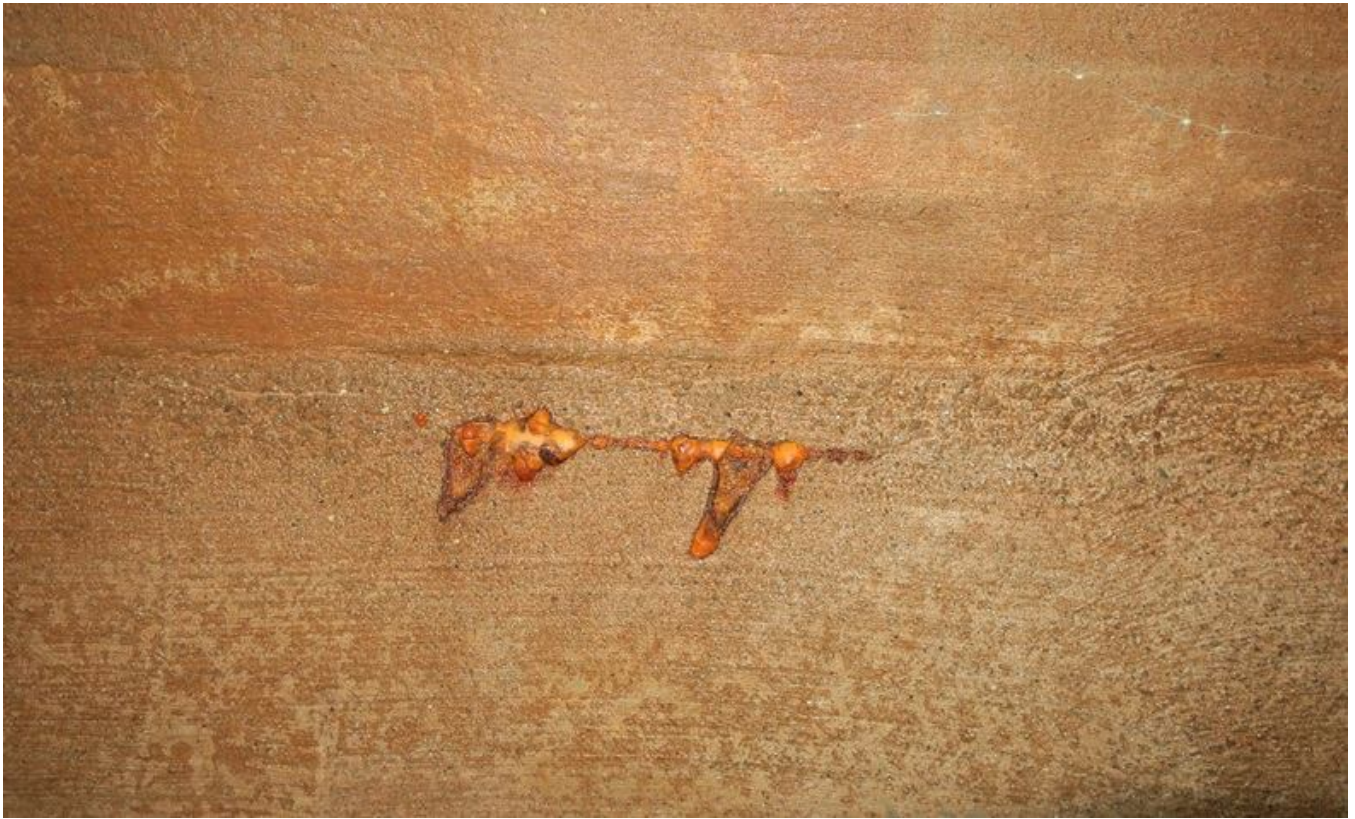
49. Rust tubercles at exposed steel in shell.
