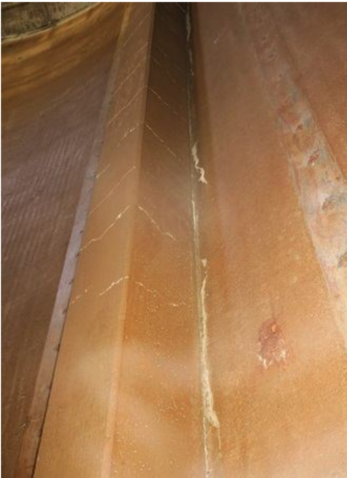
43. Concrete encasing overflow inlet.
