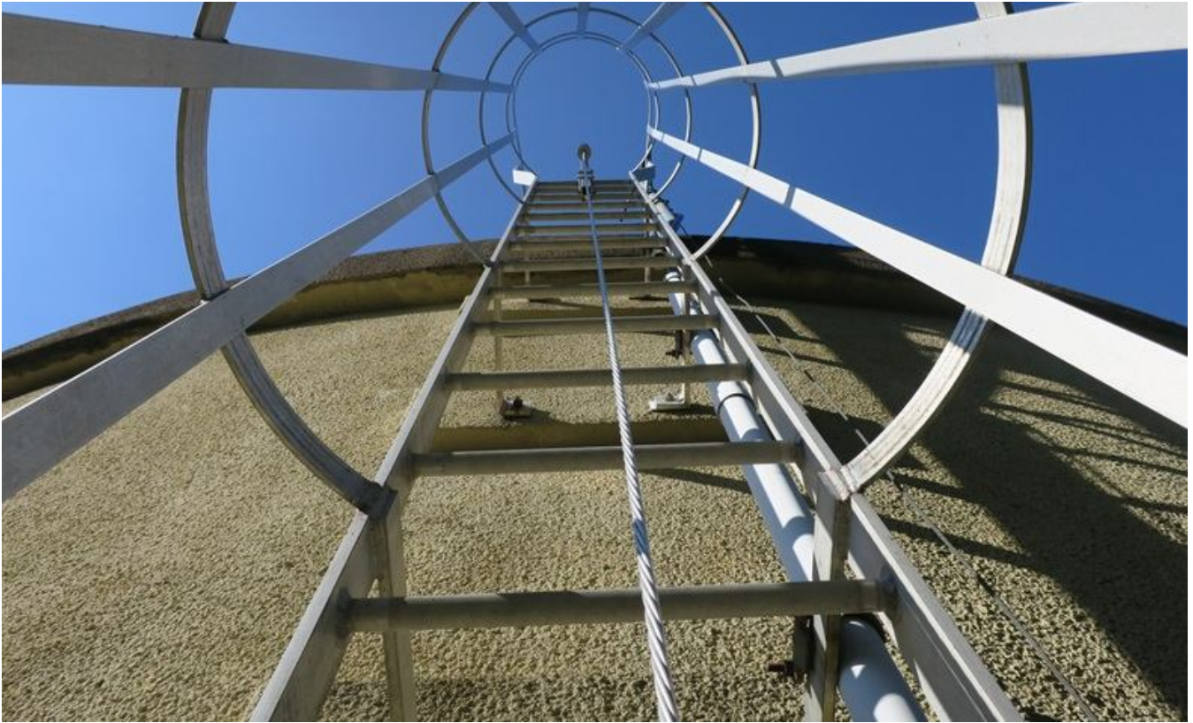
19. Exterior ladder, safety cage, and safe-climbing device.
