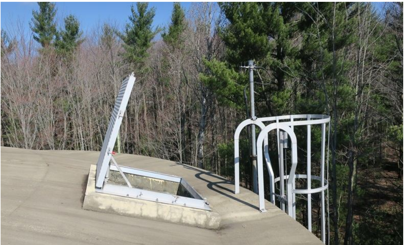
24. Roof manhole, roof access, and antenna.
