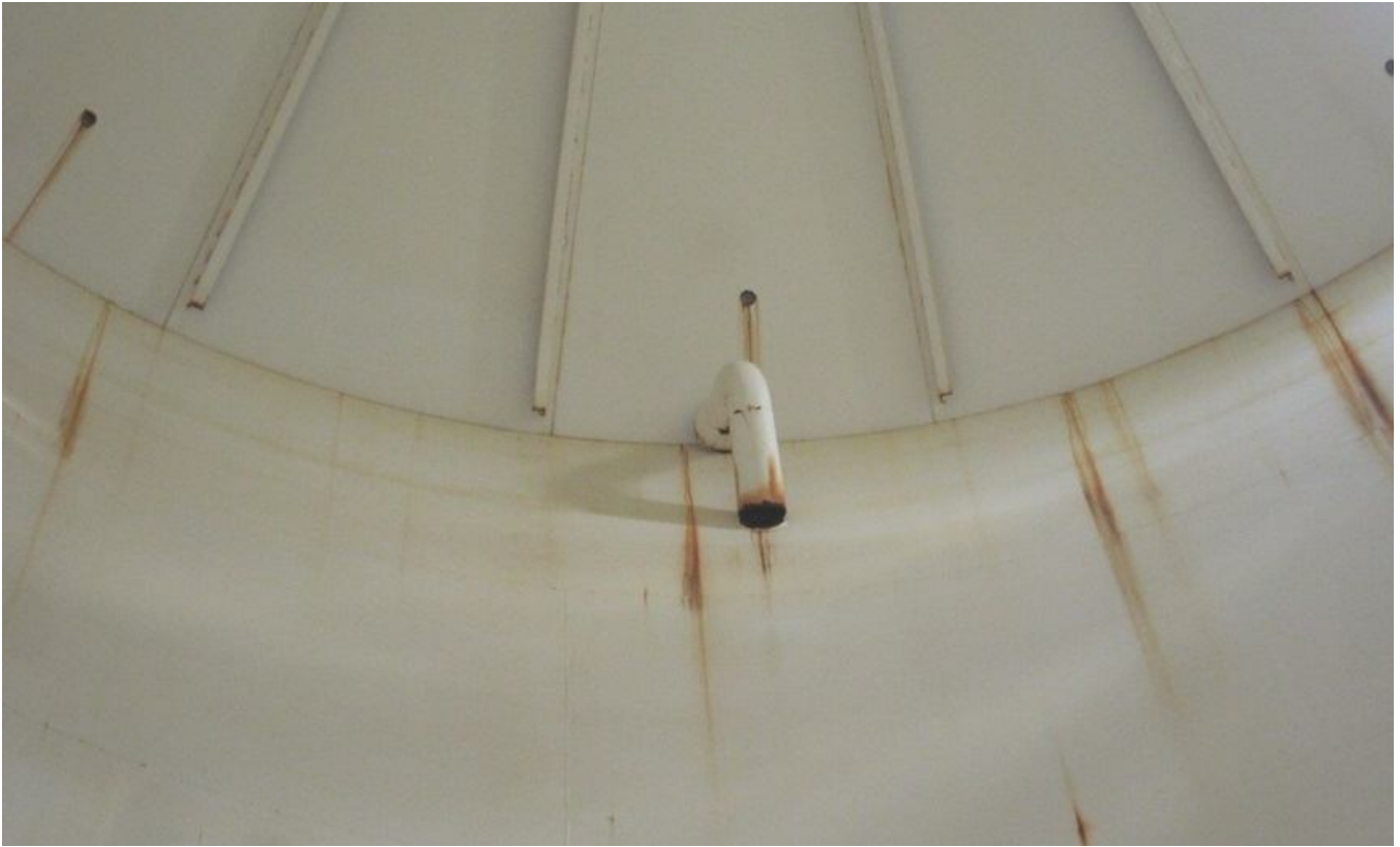
45. Overflow pipe no longer attached to shell.
