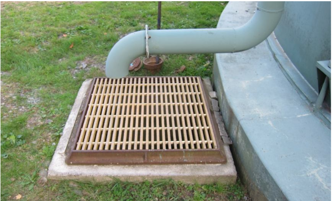
12. Overflow pipe discharge above storm drain. Note T-handle behind storm drain.
