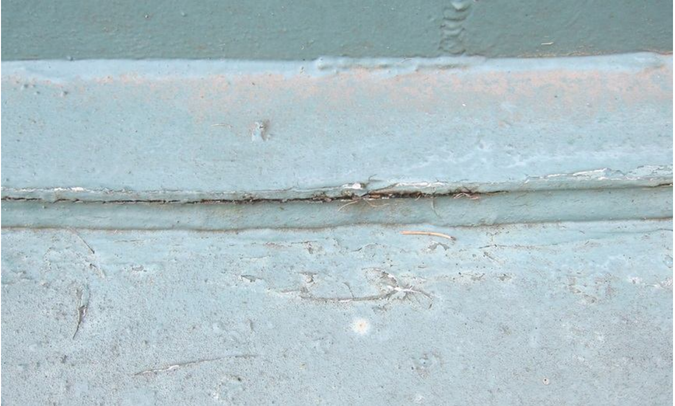
8. Tank foundation, sealant, and bottom plate projection.
