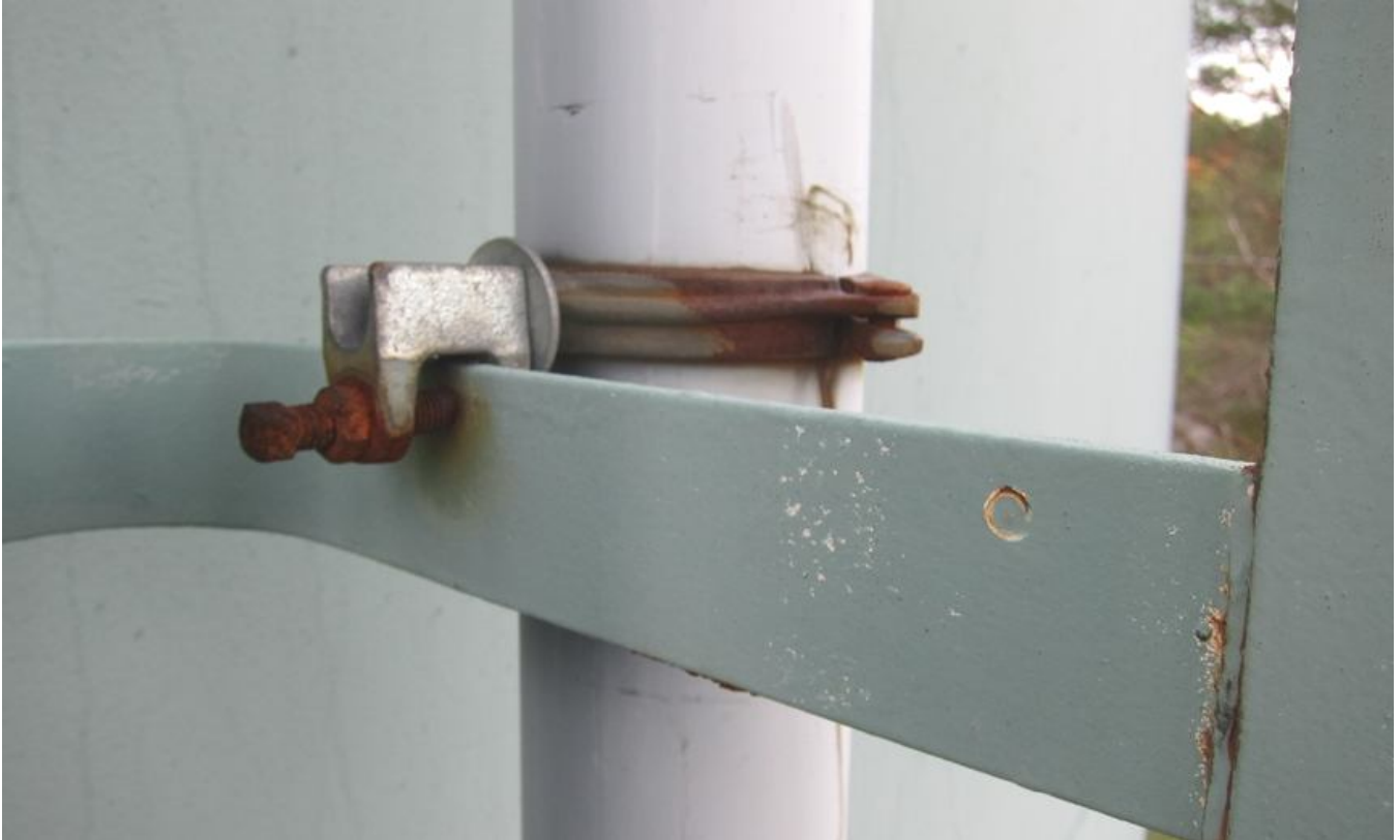
22. PVC pipe bolted to ladder safety cage.
