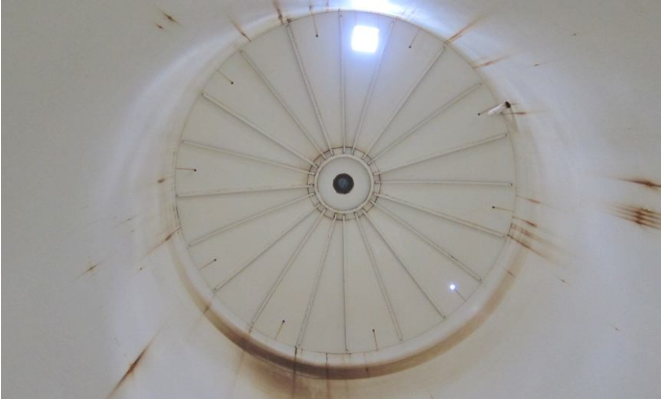
36. Roof interior and support structure.
