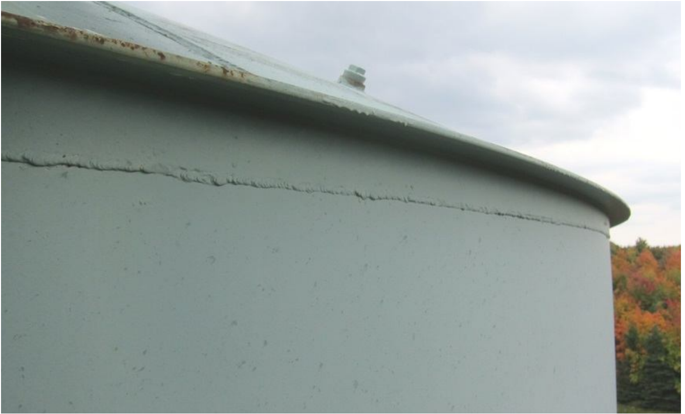
25. Top shell angle and threaded and plugged roof coupling.
