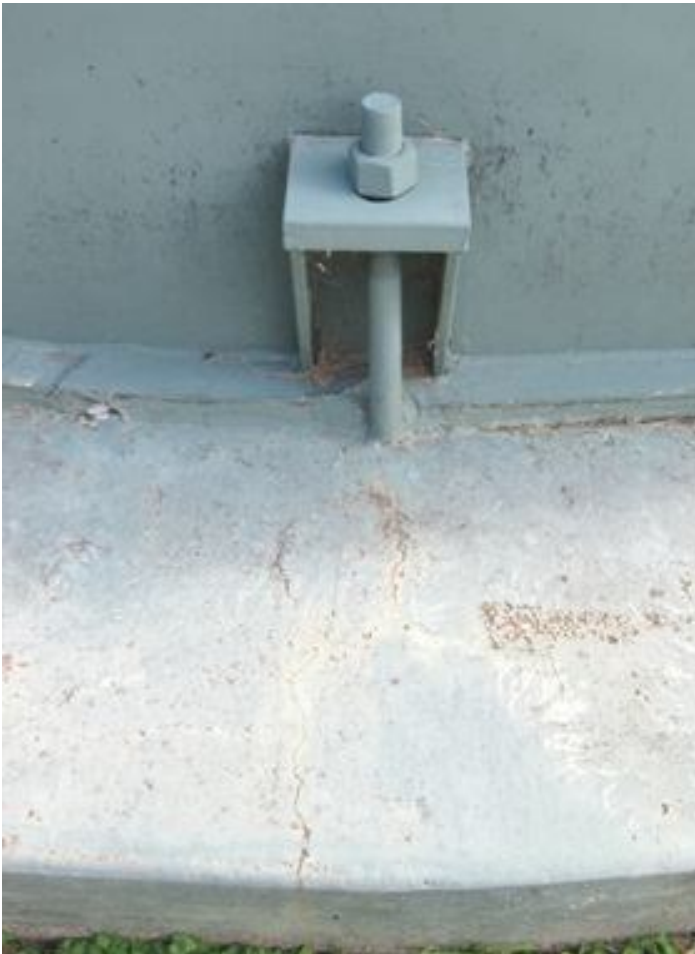
9. Tank foundation, flexible conduit, bracket, and PVC pipe.
