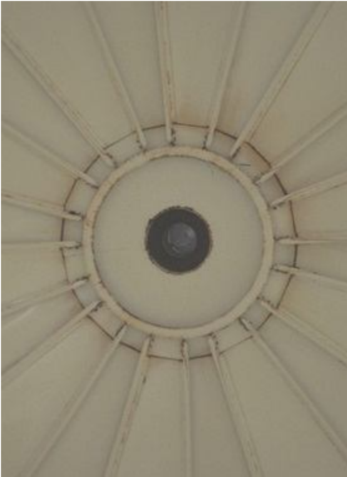
37. Roof interior and support structure.
