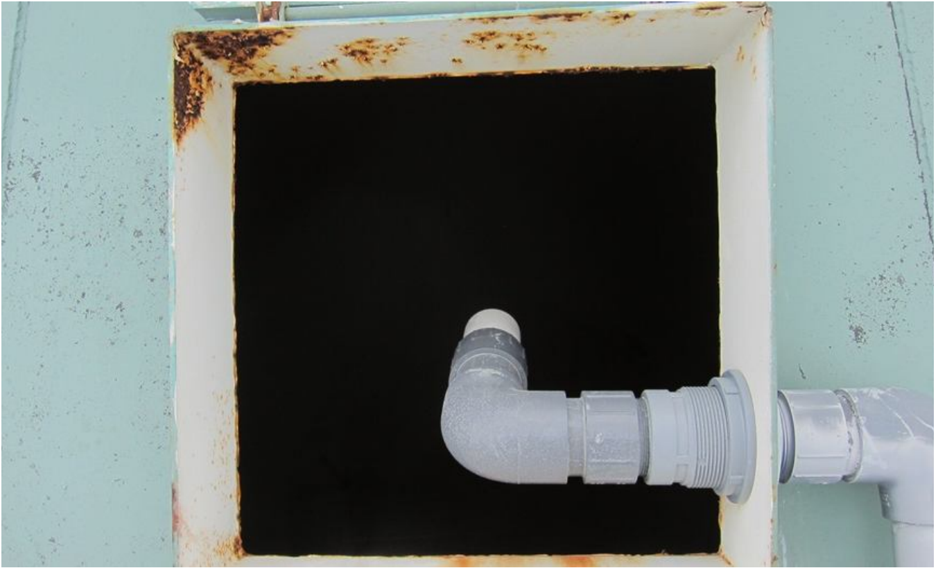
29. Piping extending into roof manhole.
