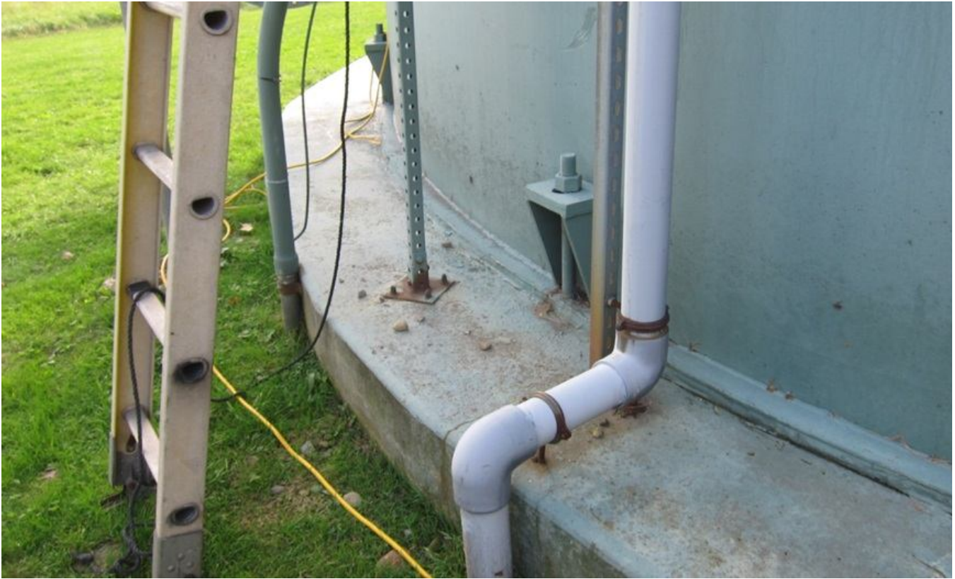
9. Tank foundation, flexible conduit, bracket, and PVC pipe.
