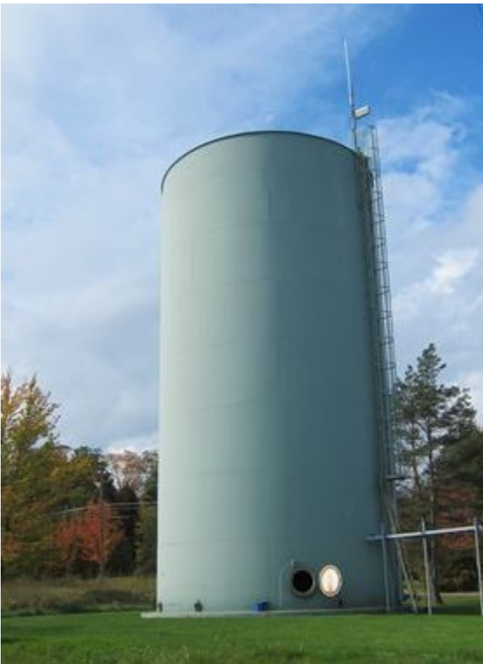
2. Tank and site.
