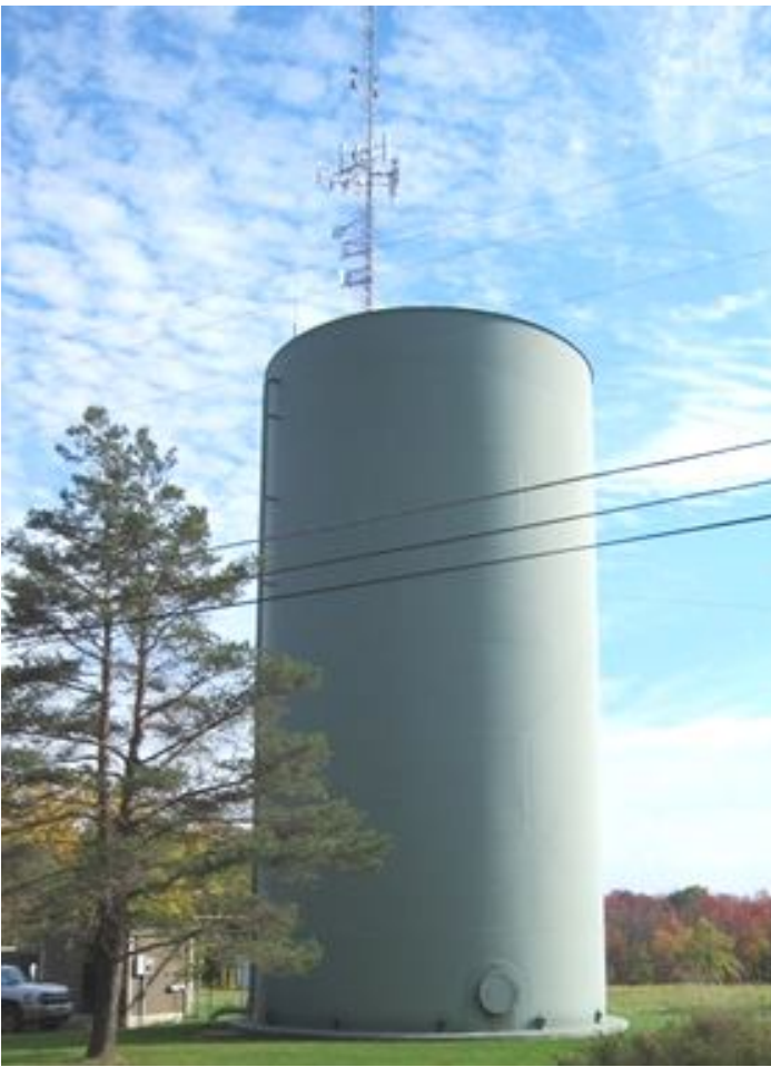
1. Tank and site.
