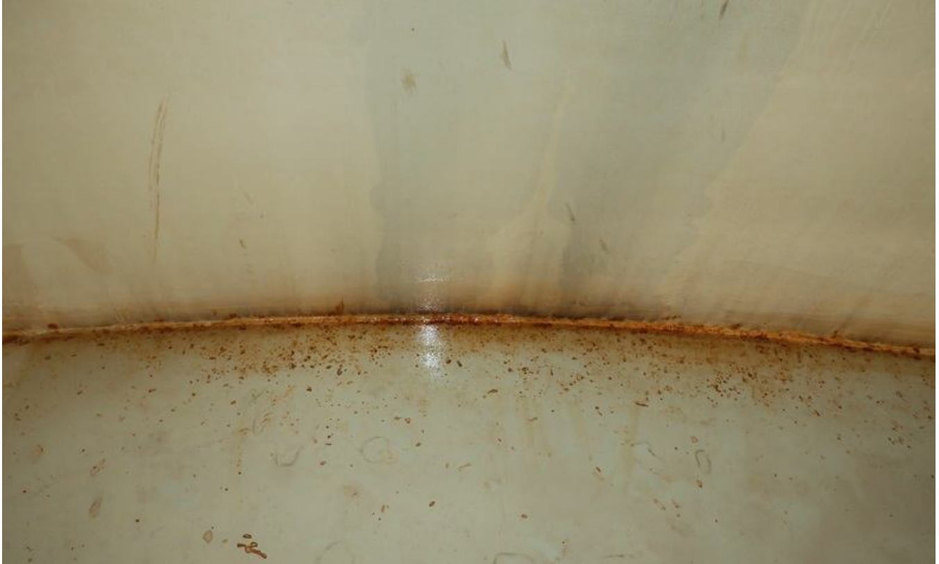
58. Interior shell and floor.
