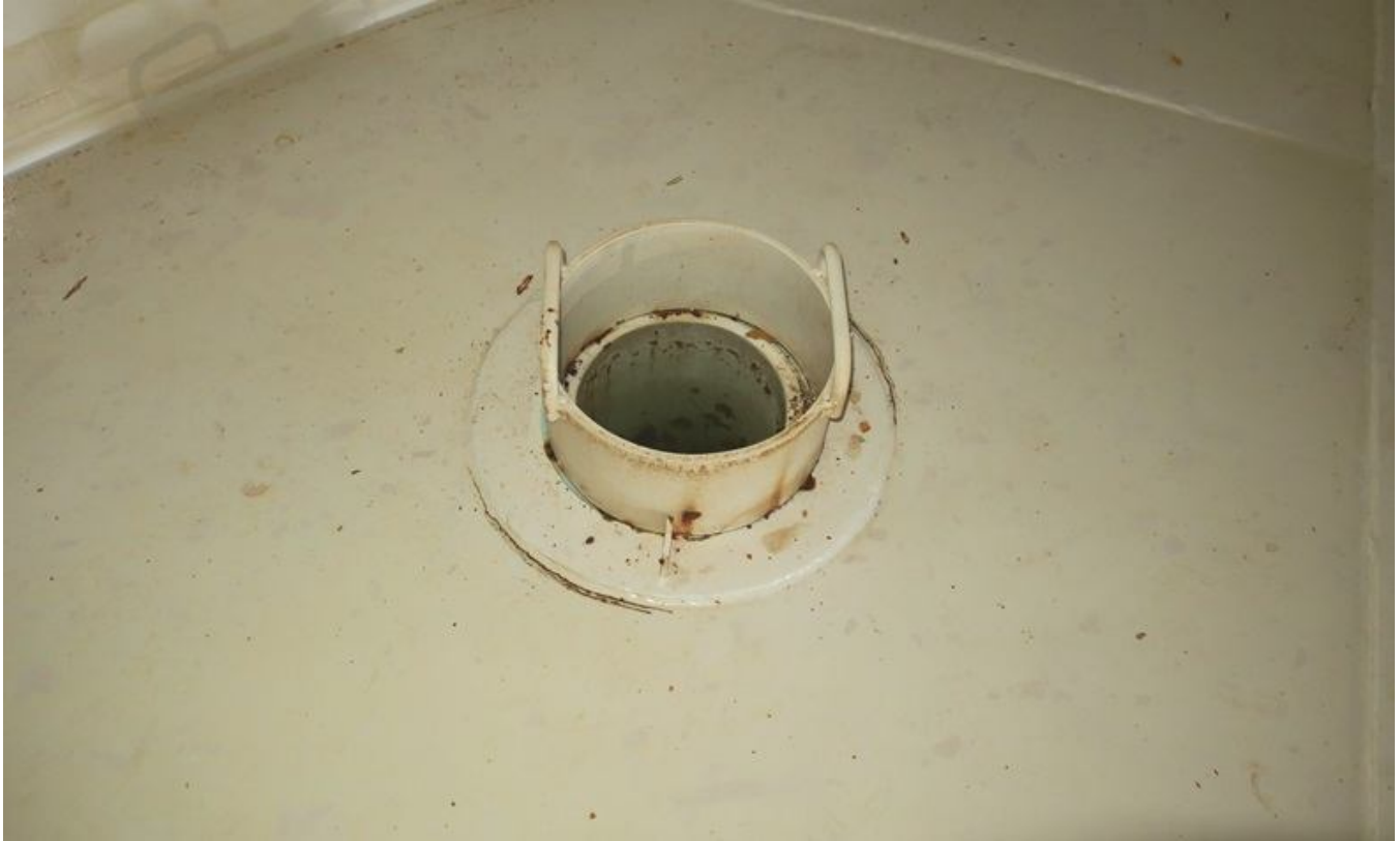
64. Outlet pipe with removable mud ring.
