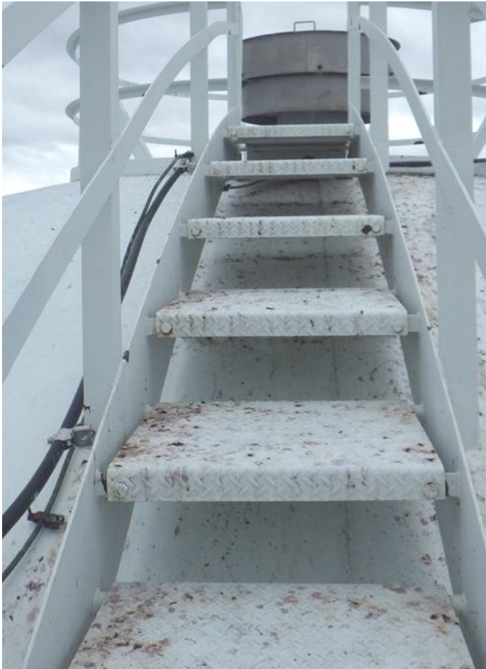
41. Stairs to roof vent.
