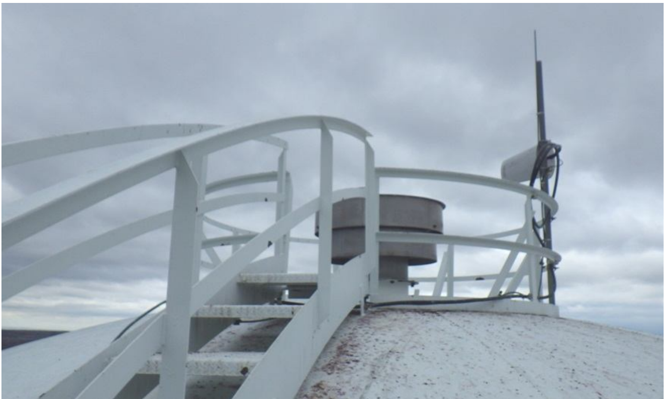
42. Stairs, railing, roof vent, and antenna.
