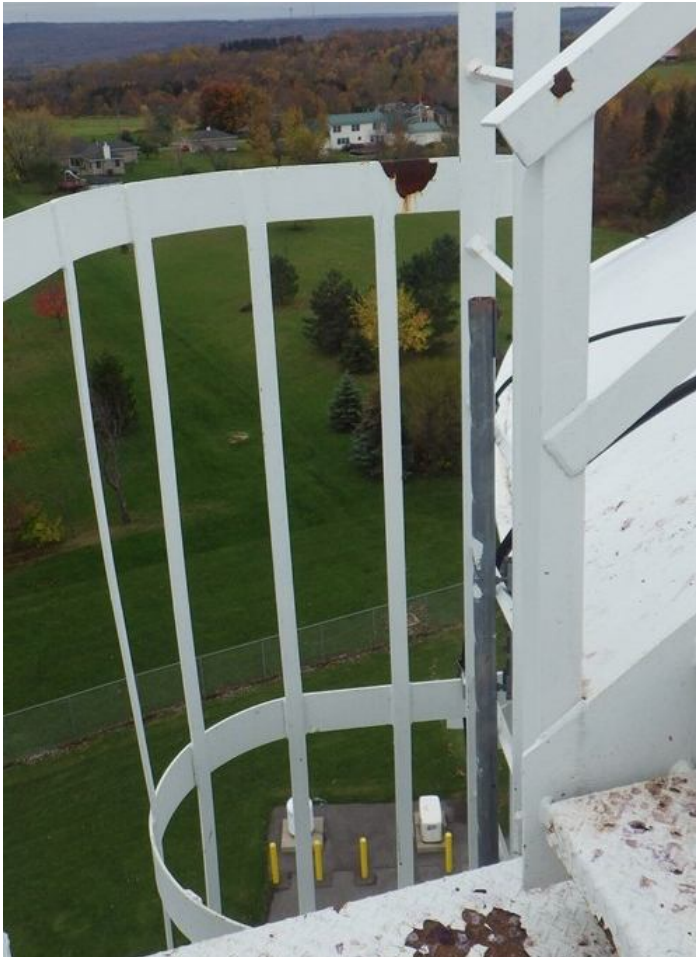
33. Shell ladder access to platform.
