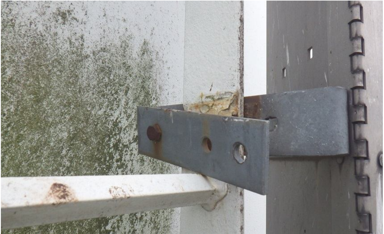
31. Unattached bracket for shell ladder vandal deterrent.
