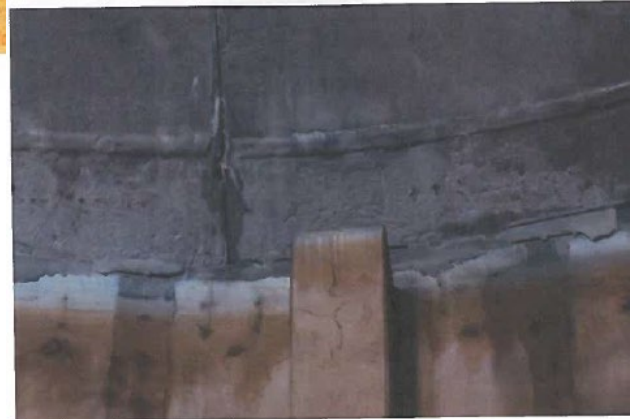
43. Concrete encasing overflow inlet.
