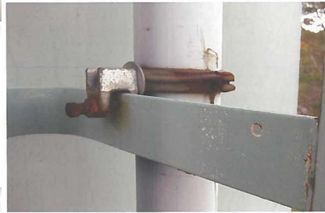
22. PVC pipe bolted to ladder safety cage.
