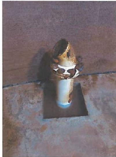
58. Corrosion on piping in sump.
