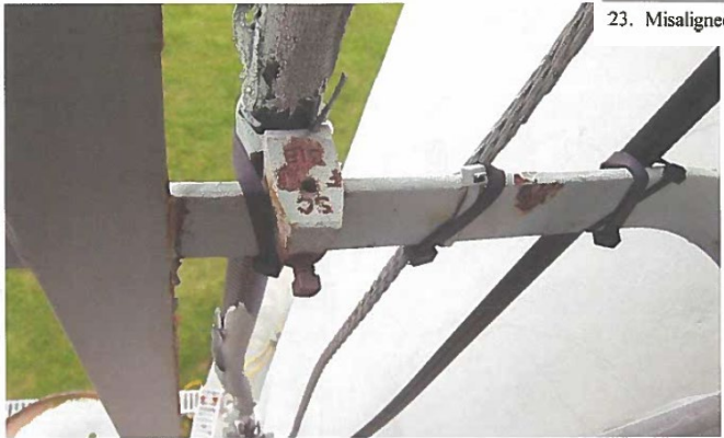
21. Flexible conduit, cable, and coaxial cable on safety cage.
