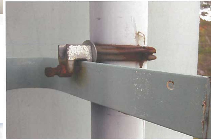
22. PVC pipe bolted to ladder safety cage.
