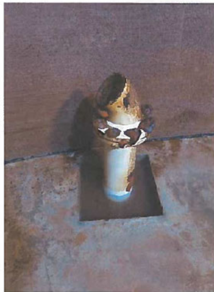
58. Corrosion on piping in sump.
