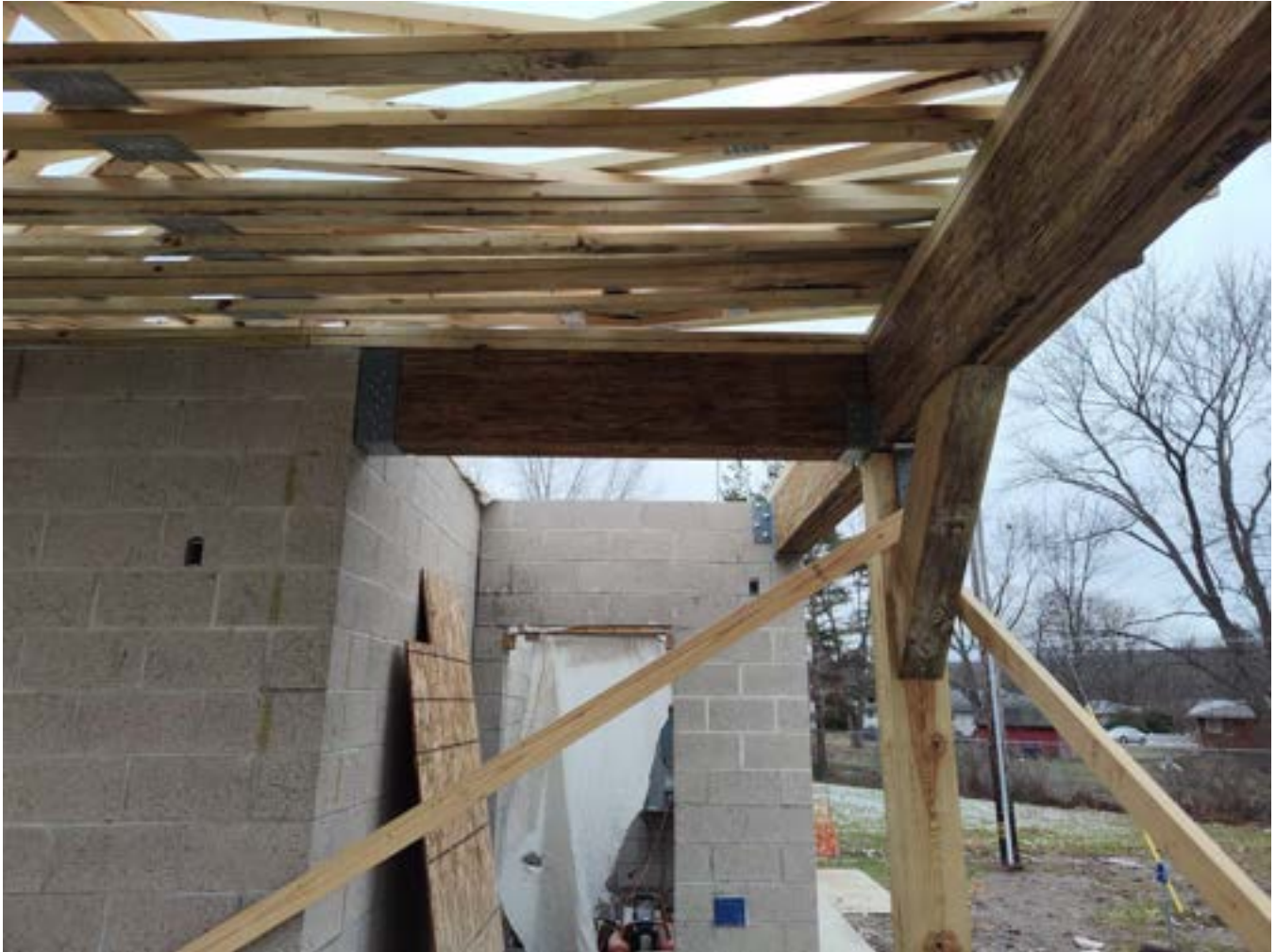
Photo 6: Wood framing connections to block building.
