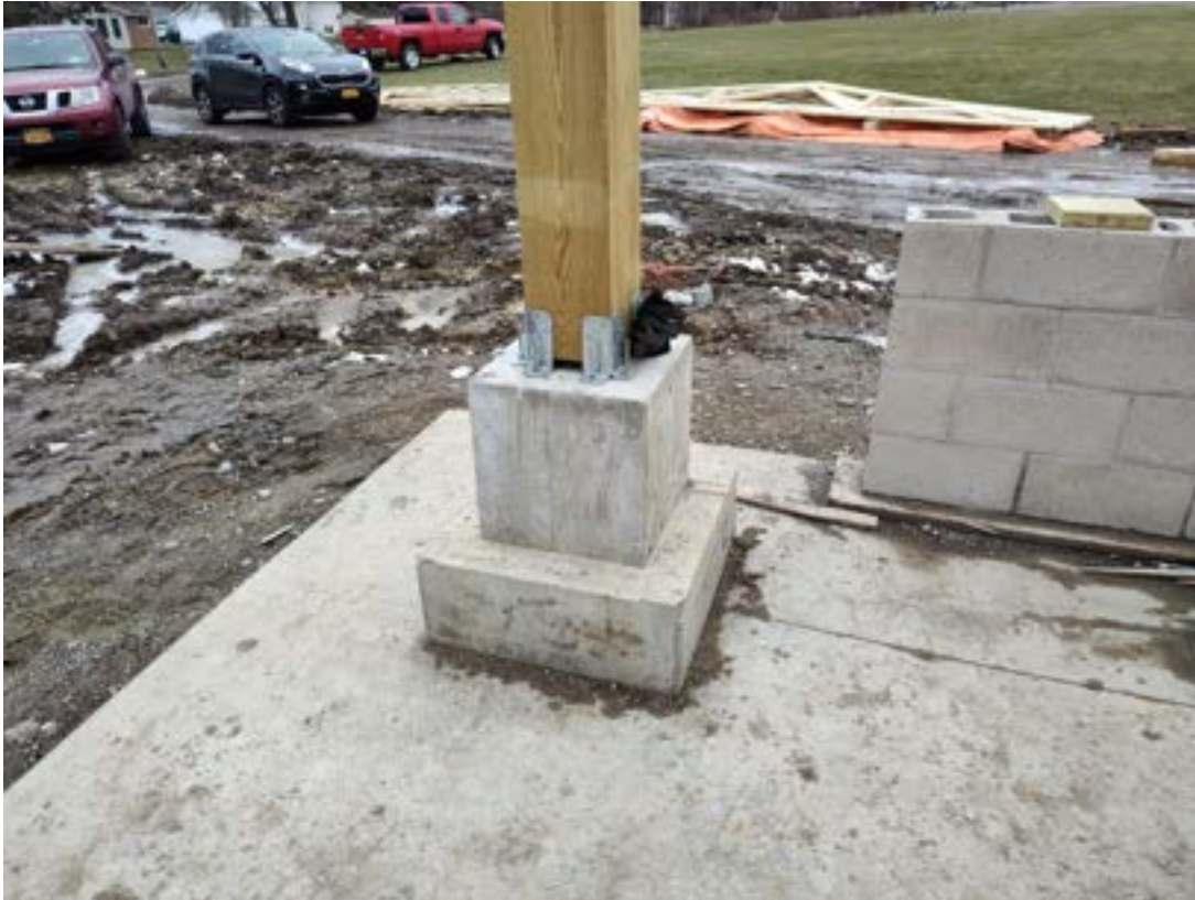
Photo 4: Wood framing and column work in progress.
