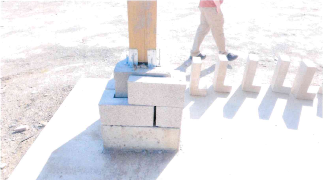
Photo 2: Mason to complete the columns, laying out blocks towards installation.
