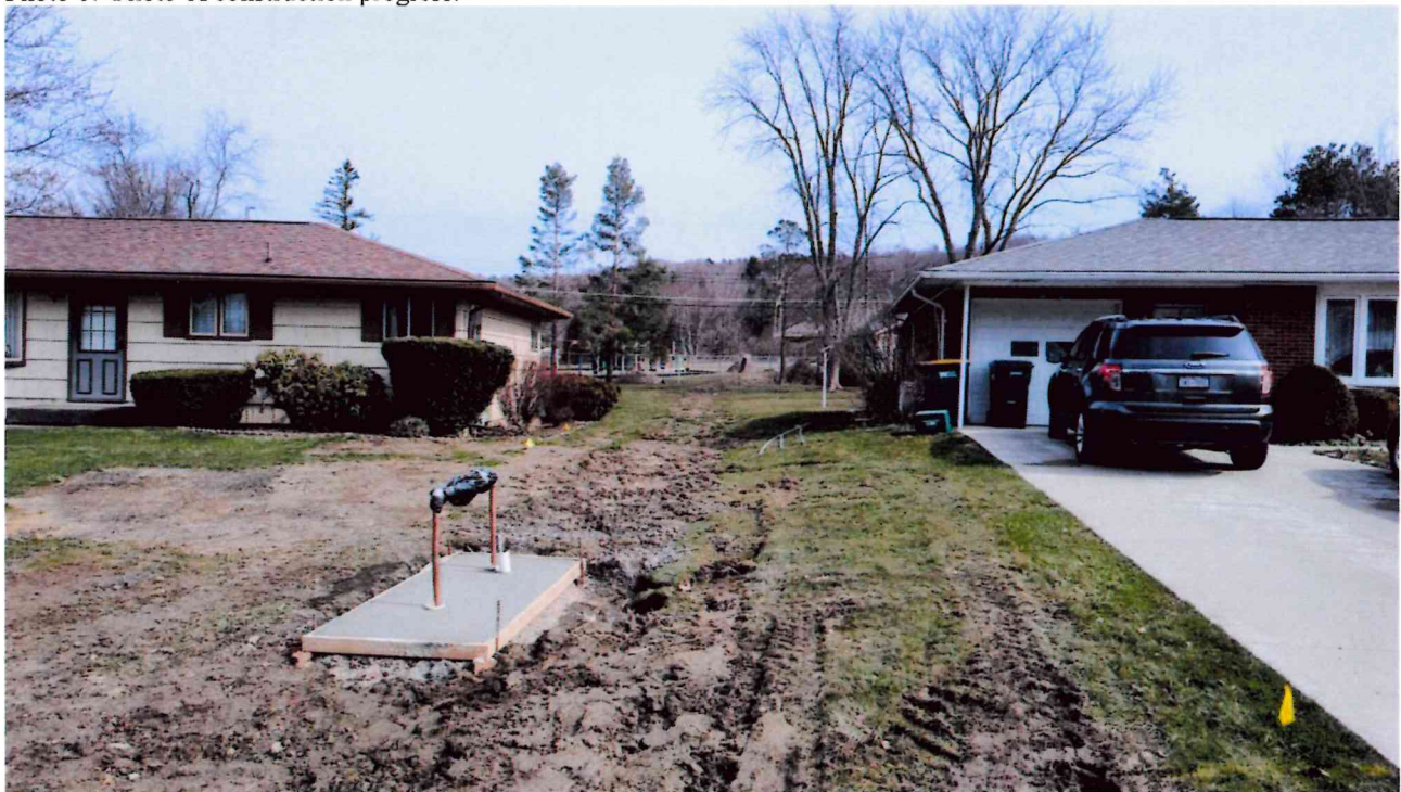
Photo 7: RPZ Concrete pad in place on Parkside.
