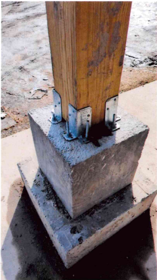
Photo 2: Mason to complete the columns.
