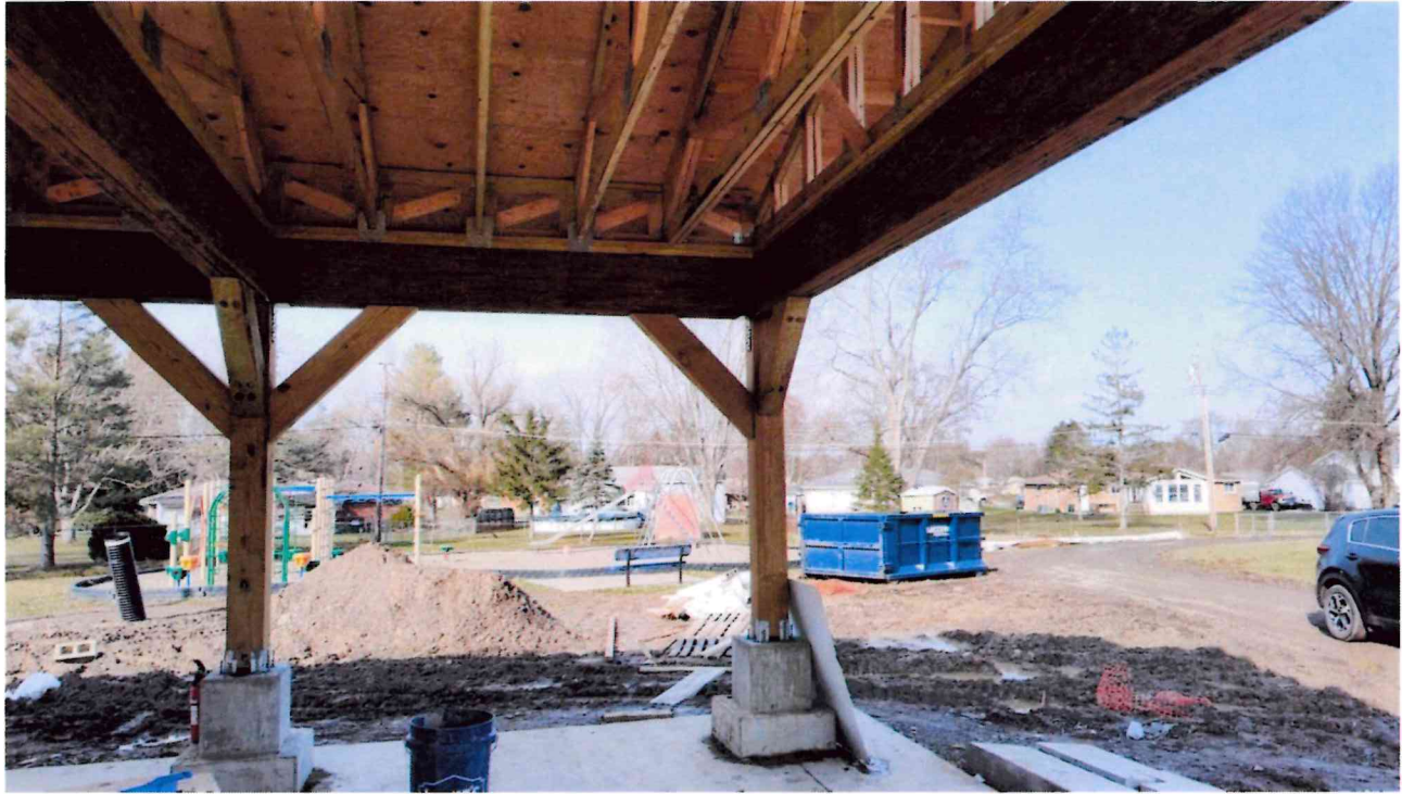
Photo 6: Photo of construction progress.
