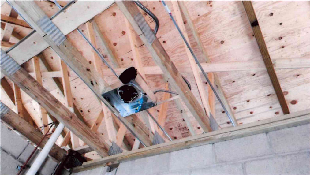
Photo 3: View of ceiling rough ins about toilet room.
