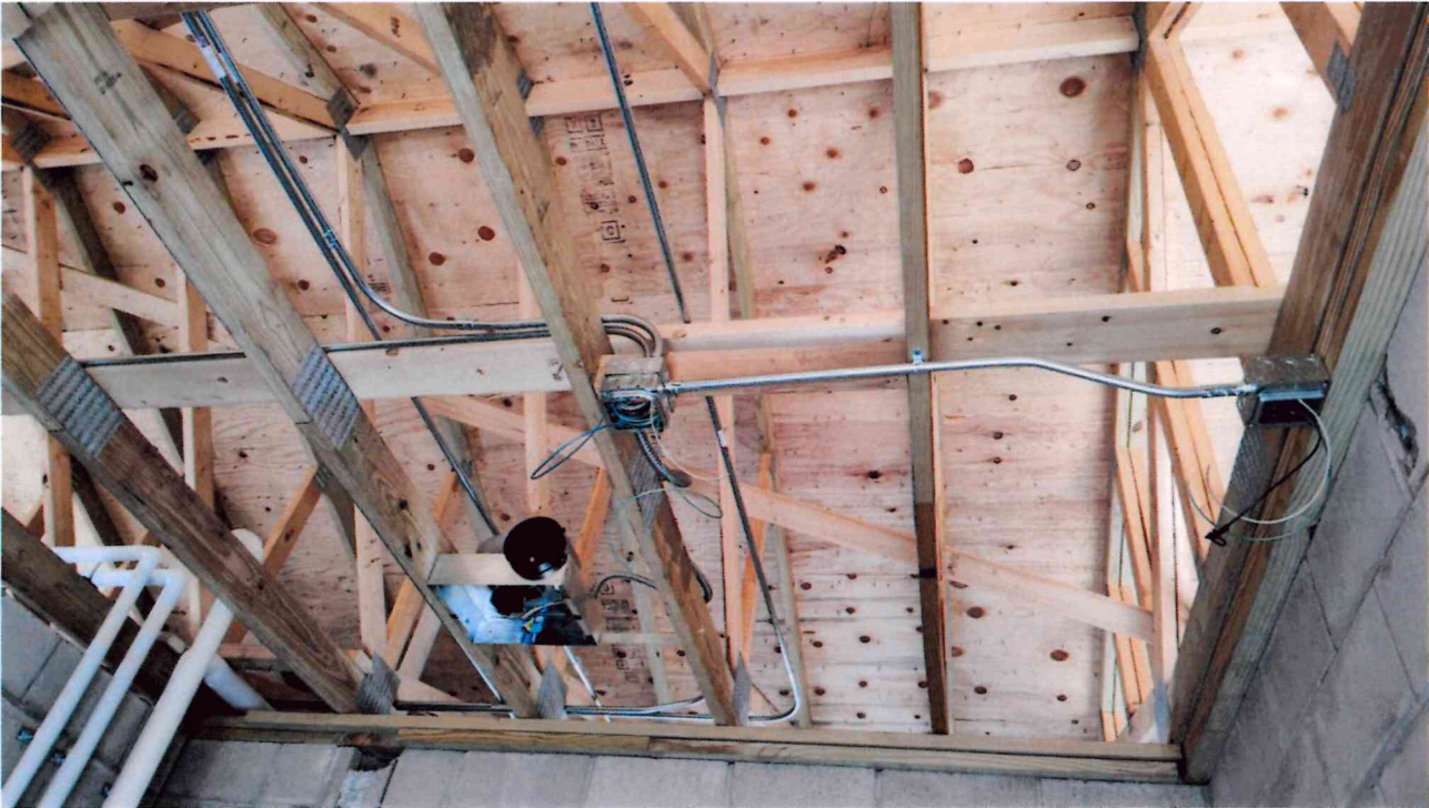
Photo 7: Photo of work in the ceiling in progress.
