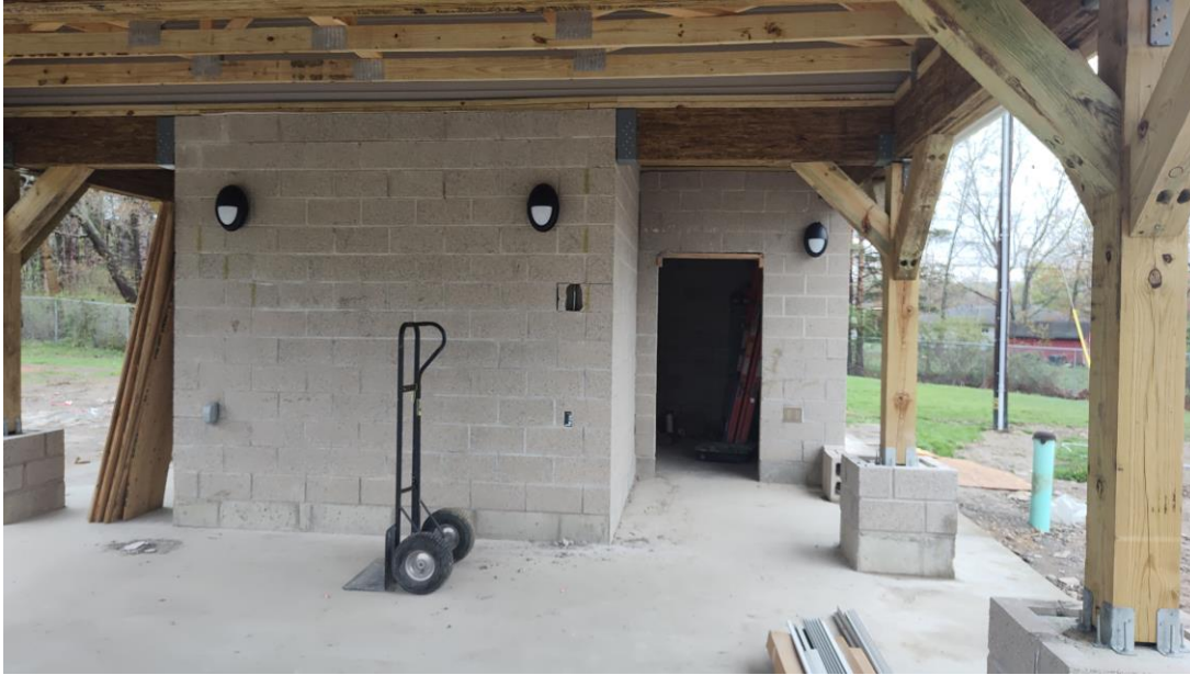
Photo 2: Exterior lighting installation.
