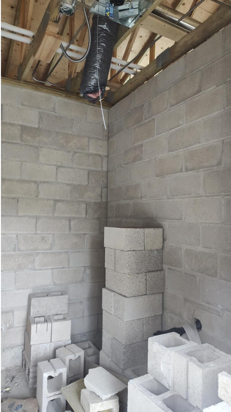
Photo 4: Block chase wall complete.
