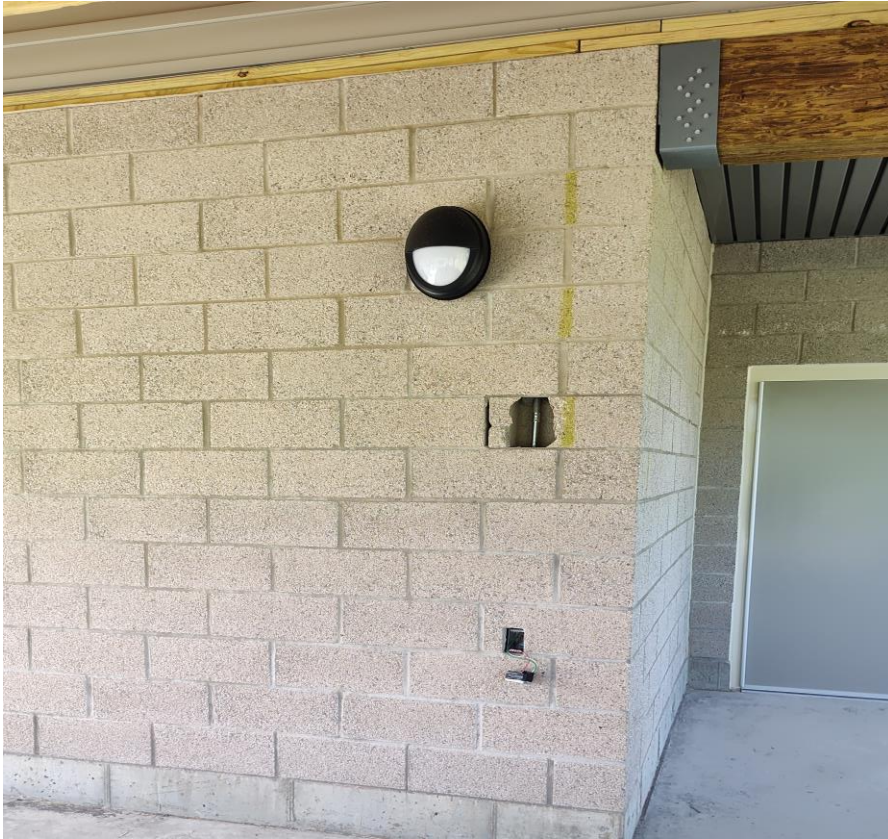
Photo 4: View of block to be replaced.
