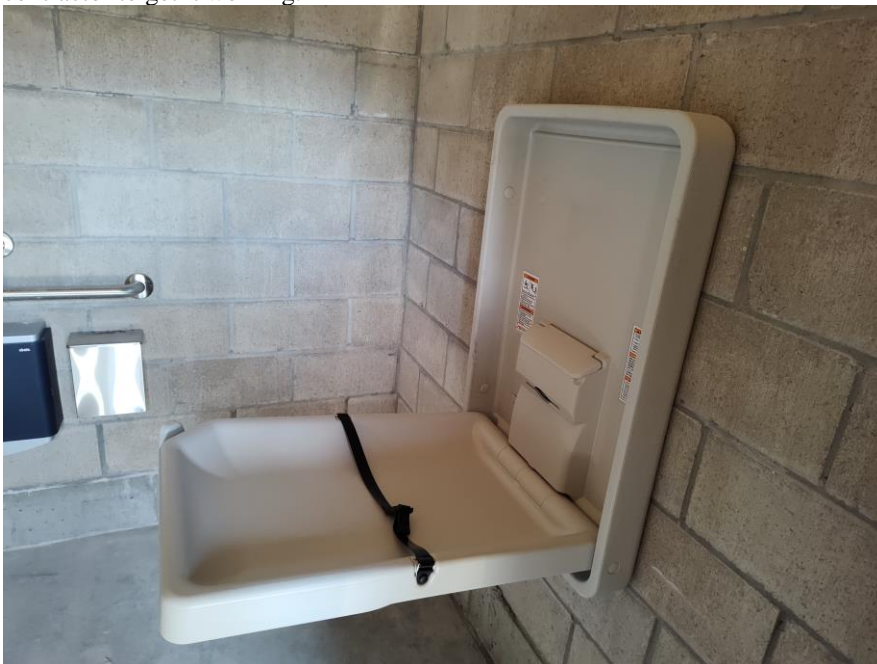
Photo 9: Changing station installed in each toilet room.
