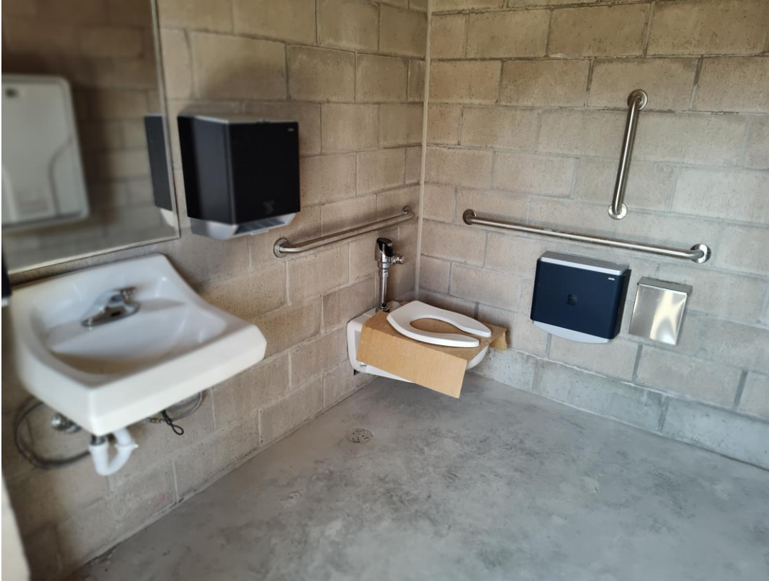
Photo 6: Plumbing fixtures installed.
