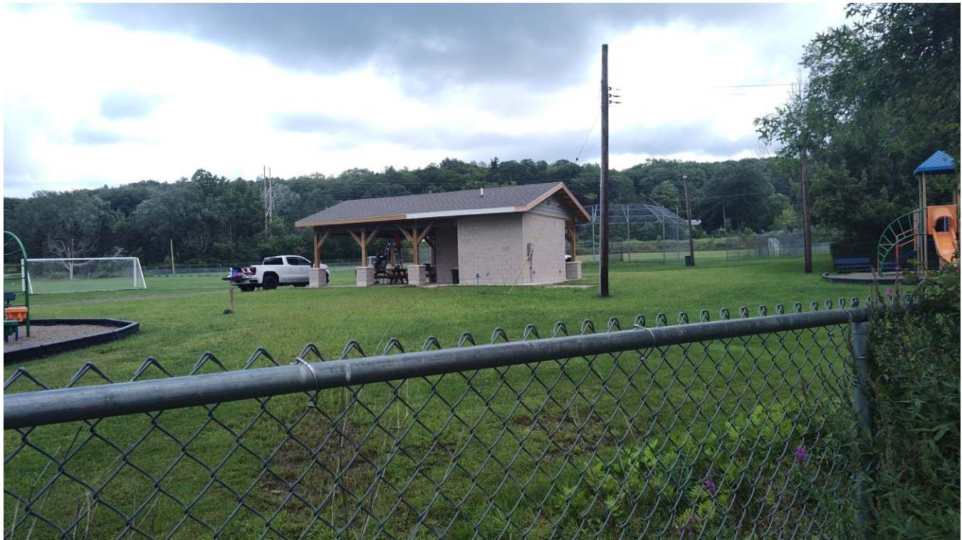
Photo 1: Photo of current site condition from Parkside backyard. Workers on site, working on the punch list items.
