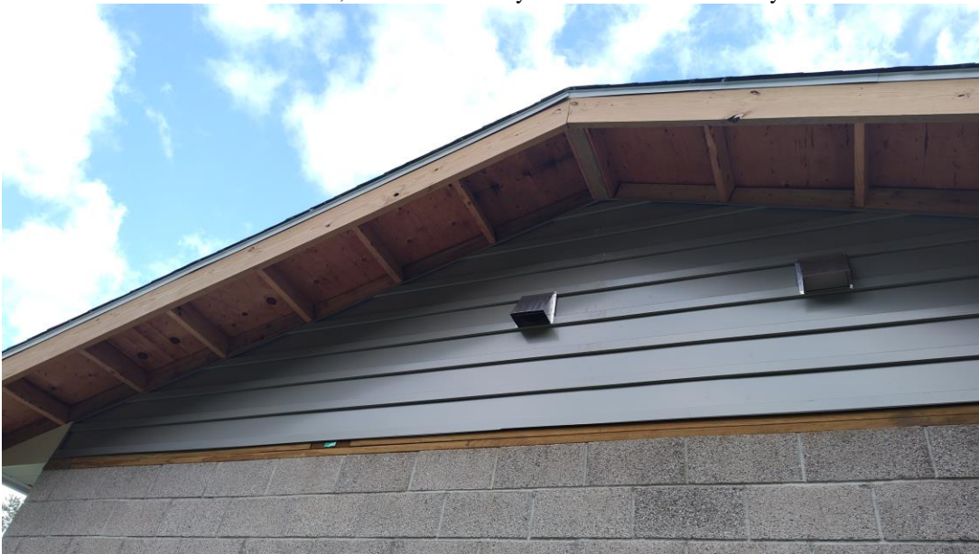
Photo 5: Also stopped on site to see the punch list items progressing. Here we see the blocking completed. Tom Tomaino fashioned a new closer piece at the ridge in this view.
