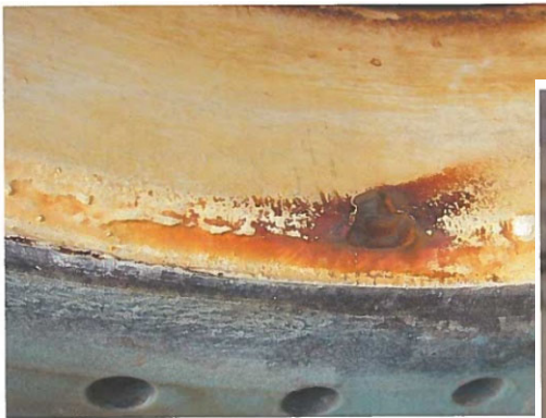
15. Corrosion and metal loss in shell manhole neck.
