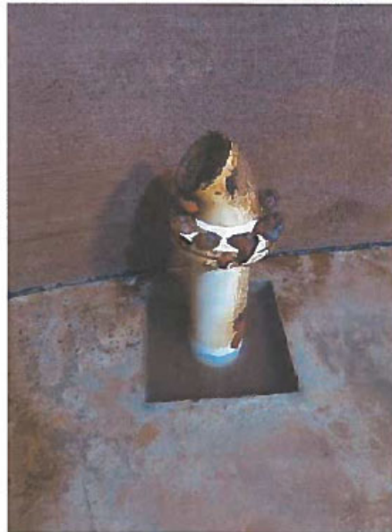
58. Corrosion on piping in sump.
