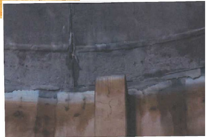
43. Concrete encasing overflow inlet.
